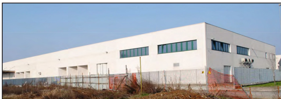
Milan Customer: Causa Pia D'Adda Maintenance works of the farms, residential and office buildings and of the Settimo Milanese Town Hall (XVI sec.).
