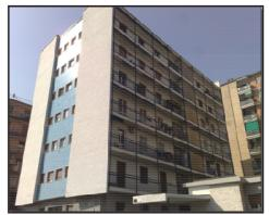
Milan, Via Palmanova, 91 Customer: Via Palmanova 91 Building, Milan, Establishment administration Repairs about two civil buildings front view. Restoration of plasters, covered in mosaic. New waterproofing for balconies and for smooth roof. Finishing touches and painting works. Involved surfaces: Flat covering about 1,400.00 m<sup>2</sup> Balconies flooring about 800 m<sup>2</sup> Front views about 4,800.00 m<sup>2</sup>
