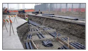
**Milan - Customer: Sirti S.p.A.**Excavations and reinstatement to set down four parallel power lines at Milan building site - via Barzaghi.
